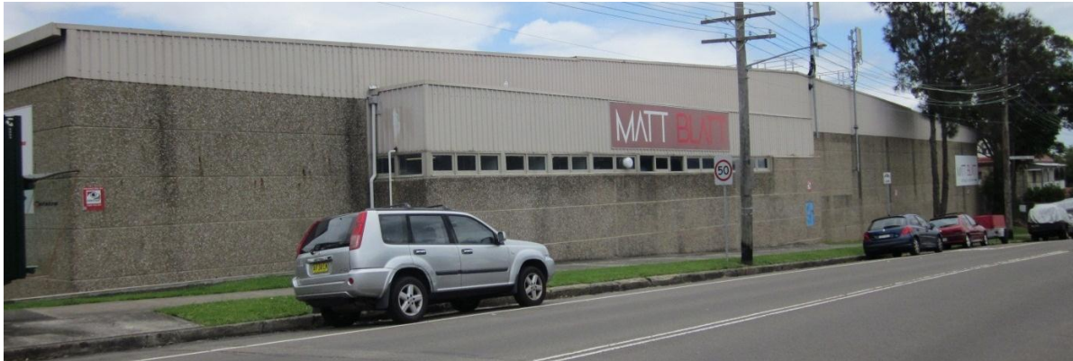
Figure 4: 141 Allen Street – Looking north east from the intersection of Flood Street & Allen Street (Flood Street Elevation)
