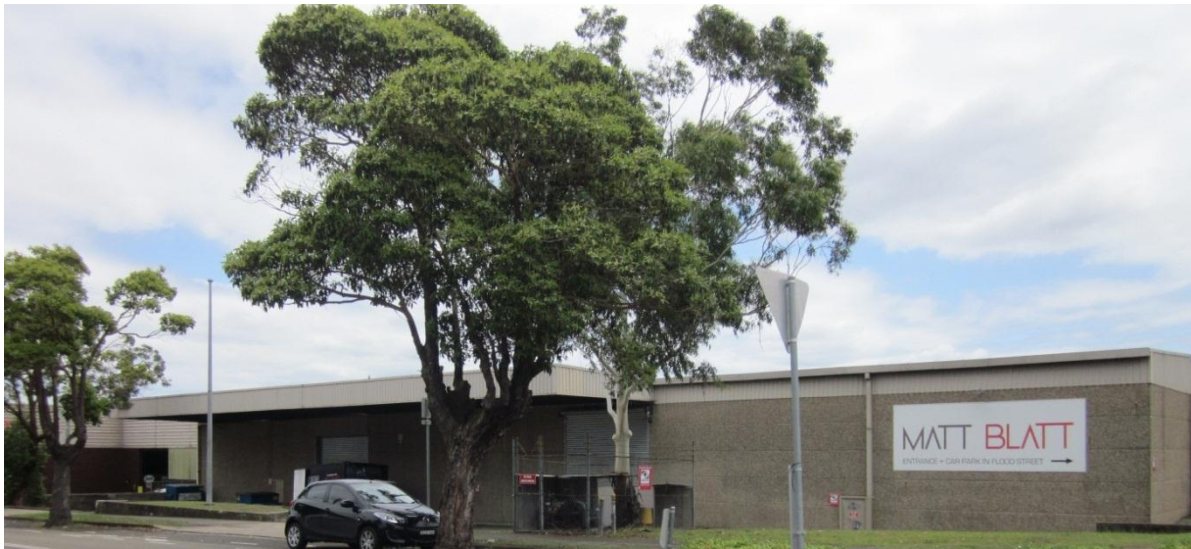
Figure 5: 141 Allen Street – Flood Street frontage looking northwest
